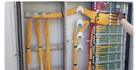
Fiber Backbone Distribution
